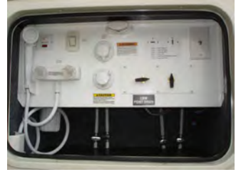
Fig. B - Utility Center
